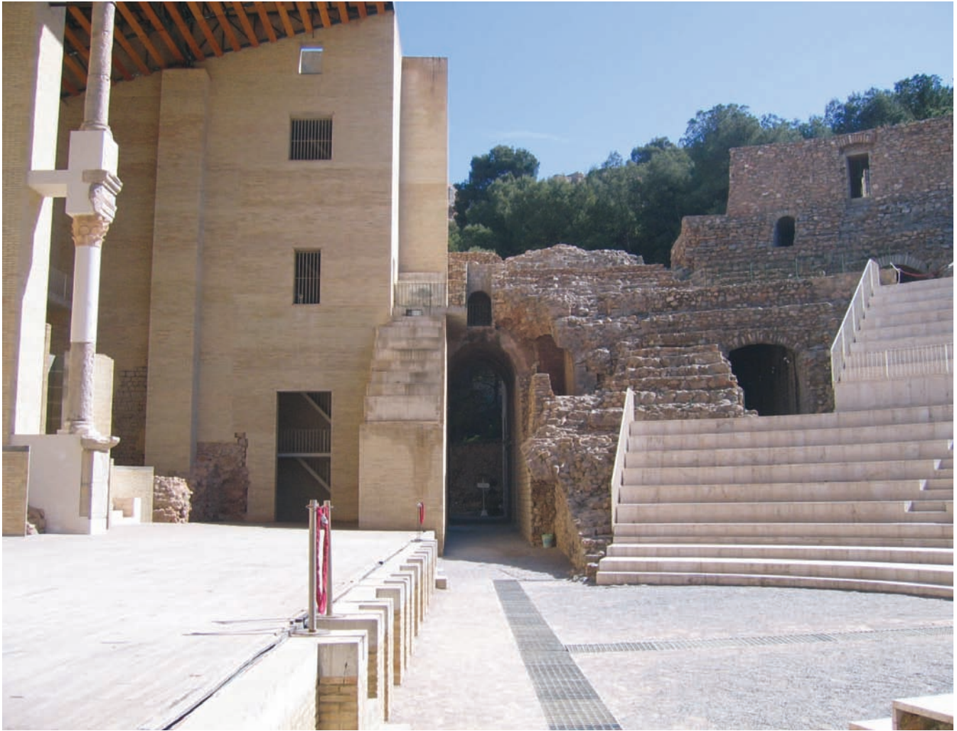
Figure 9. The rehabilitated Sagunt theatre.
